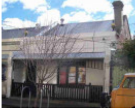
fitzroy argyle street fitzroy argyle street 111
