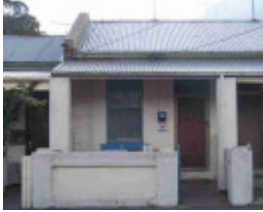
fitzroy argyle street fitzroy argyle street 167
