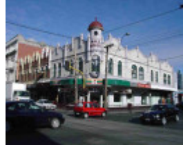
Fitzroy Brunswick Street 287- 295.JPG
