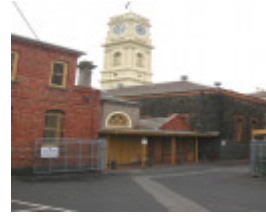
Prahran Town Hall South Elevation 2 May 05
