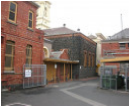
Prahran Town Hall South Elevation 3 May 05
