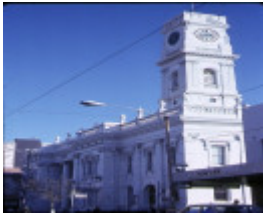
h00203 prahran town hall prahran exterior view
