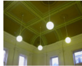
h00203 prahran town hall interior first town hall 2 may05
