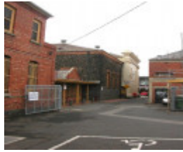
Prahran Town Hall South Elevation 4 May 05
