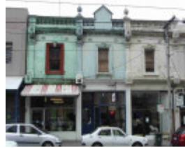
Fitzroy Brunswick Street 83- 87.JPG
