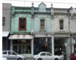
Fitzroy Brunswick Street 83- 87.JPG
