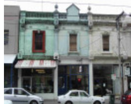
Fitzroy Brunswick Street 83- 87.JPG
