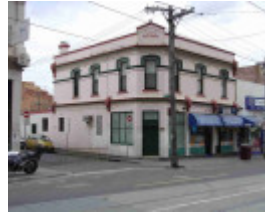
Fitzroy Brunswick Street 99- 103.JPG
