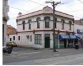
Fitzroy Brunswick Street 99- 103.JPG
