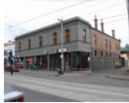
Fitzroy Brunswick Street 109- 115.JPG
