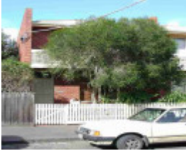
fitzroy fitzroy street fitzroy fitzroy street 322 unit 1
