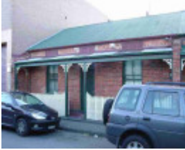
fitzroy chapel street fitzroy chapel street 7
