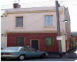
fitzroy kerr street fitzroy kerr street 81
