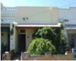
fitzroy north bennett street fitzroy north bennett street 36
