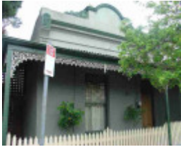
fitzroy north coleman street fitzroy north coleman street 19
