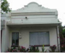
fitzroy north coleman street fitzroy north coleman street 26
