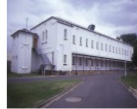
mayday hills hospital albert street beechworth rear view dec1984
