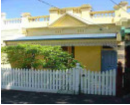
fitzroy north bennett street fitzroy north bennett street 31
