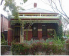
fitzroy north brennand street fitzroy north brennand street 2
