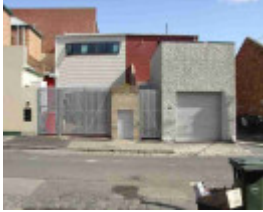
fitzroy fitzroy street fitzroy fitzroy street 101 unit 1
