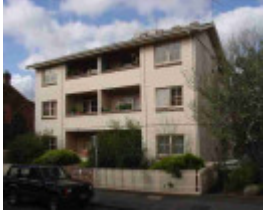
fitzroy fitzroy street fitzroy fitzroy street 170-176 unit 1
