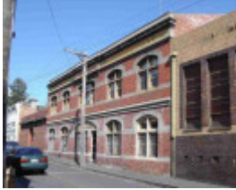
fitzroy fitzroy street fitzroy fitzroy street 175 unit 1
