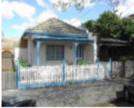
fitzroy kerr street fitzroy kerr street 46
