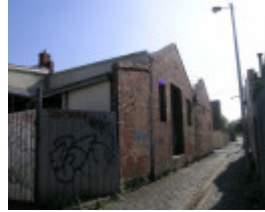
Rear of 428 Brunswick Street.JPG
