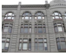
Elaborate detailing on the eastern face
