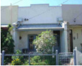
fitzroy north bennett street fitzroy north bennett street 34
