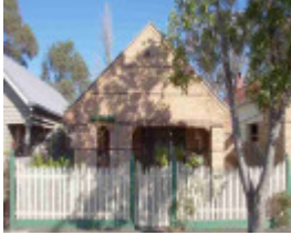
clifton hill walker street clifton hill walker street 69
