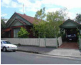
clifton hill spensley street clifton hill spensley street 32 unit c
