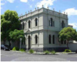
richmond docker street richmond docker street 37
