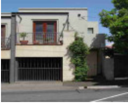
richmond docker street richmond docker street 46
