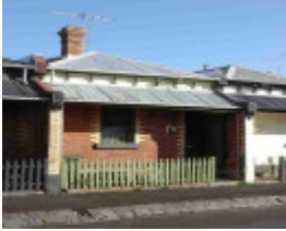
fitzroy garfield street fitzroy garfield street 8
