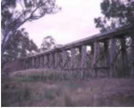
1 rail bridge over hansford creek pyalong side elevation apr 95
