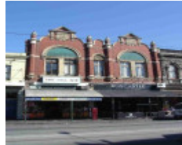
Fitzroy Brunswick Street 337- 339.JPG
