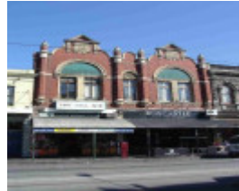
Fitzroy Brunswick Street 337- 339.JPG
