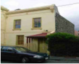
fitzroy hodgson street fitzroy hodgson street 23
