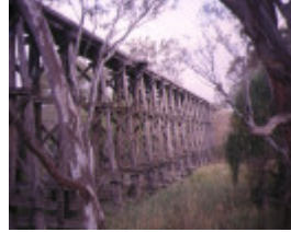
1 rail bridge over mollisons creek pyalong side elevation apr1995
