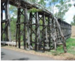
RAIL BRIDGE SOHE 2008
