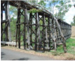
RAIL BRIDGE SOHE 2008
