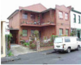
fitzroy james street fitzroy james street 5
