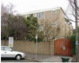
Fitzroy Napier Street 35-41 Unit 1-24 part.JPG
