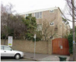
Fitzroy Napier Street 35-41 Unit 1-24 part.JPG
