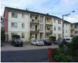
fitzroy condell street fitzroy condell street 60 unit 1-9
