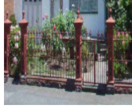
Fence - 417 Canning Street
