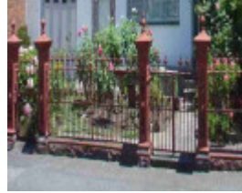
Fence - 417 Canning Street
