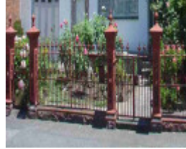
Fence - 417 Canning Street
