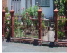
Fence - 417 Canning Street
