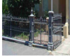
Fence - 419 Canning Street
