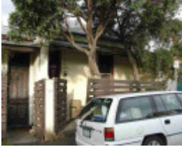
fitzroy elliot street fitzroy elliot street 3
