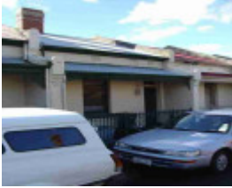
fitzroy garfield street fitzroy garfield street 5
