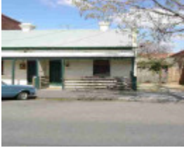
fitzroy kerr street fitzroy kerr street 54
