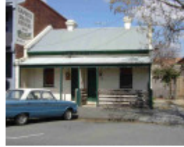
Fitzroy Kerr Street 54-56.JPG
