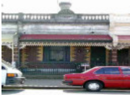
fitzroy kerr street fitzroy kerr street 61
