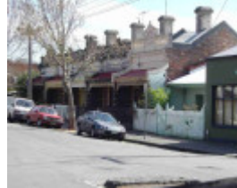
Fitzroy Kerr Street 55-63.JPG
