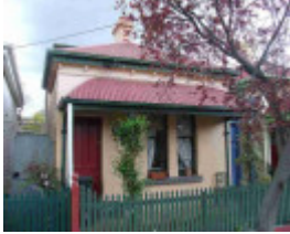
fitzroy north egremont street fitzroy north egremont street 11
