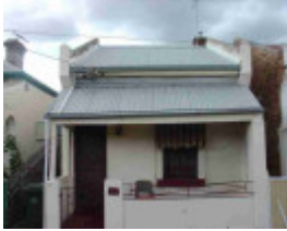
fitzroy north egremont street fitzroy north egremont street 12
