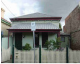
fitzroy north egremont street fitzroy north egremont street 15
