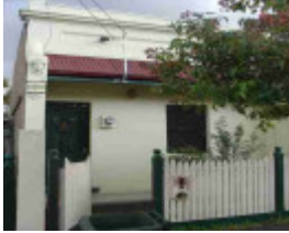
fitzroy north egremont street fitzroy north egremont street 17
