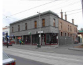
Fitzroy Brunswick Street 109- 115.JPG
