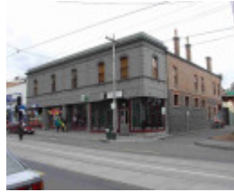
Fitzroy Brunswick Street 109- 115.JPG
